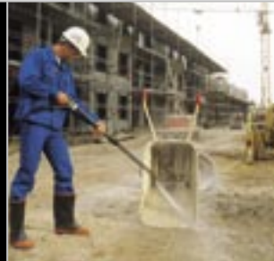
Maintenance with high pressure
